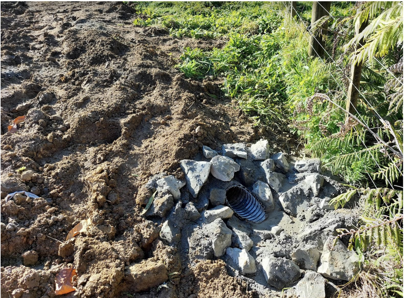
Underfill drain outlets at Lot 950 and 949
