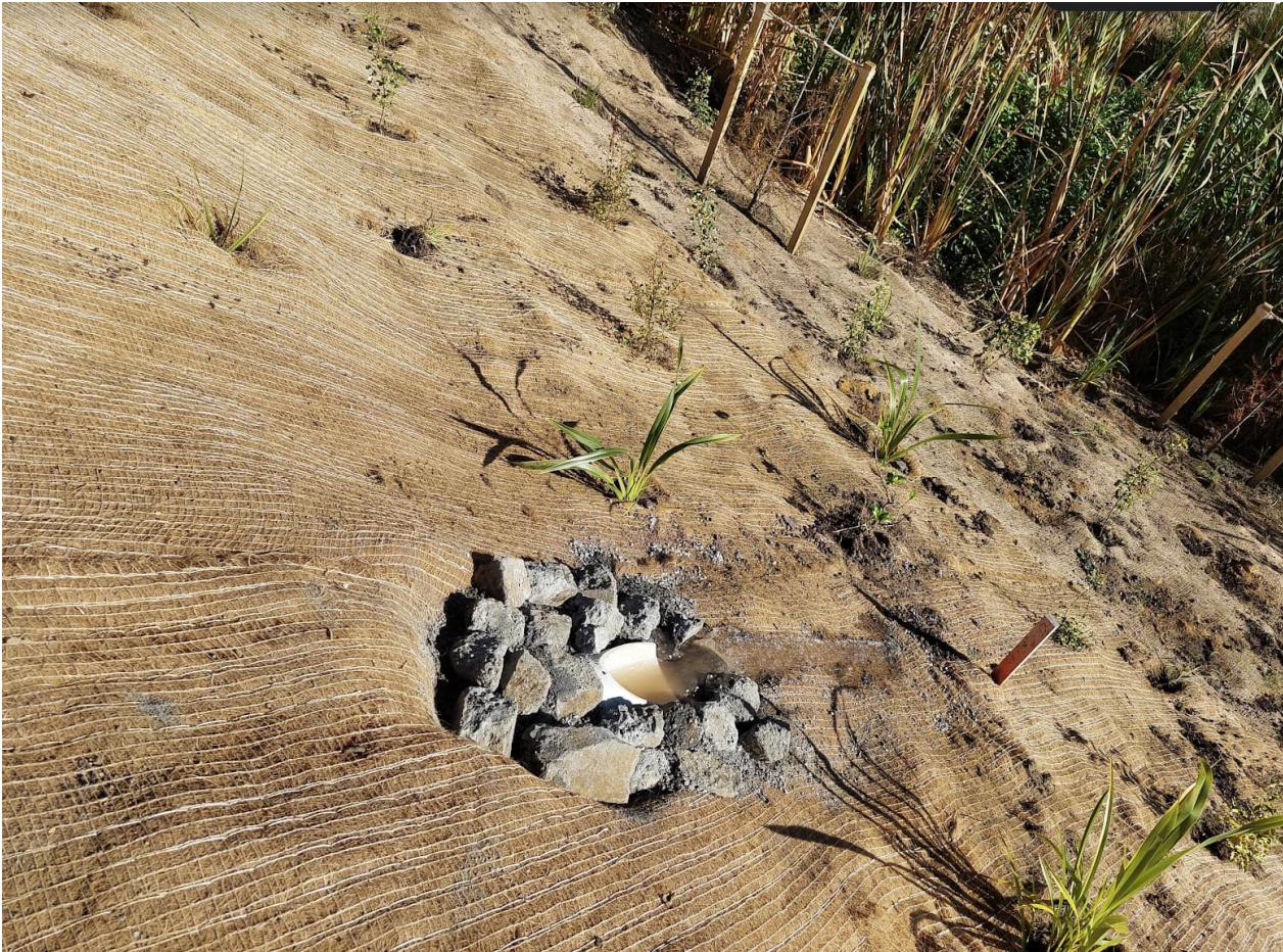
Contractor exposed underfill drain (toe of REB1) that was previously covered in vege mat
