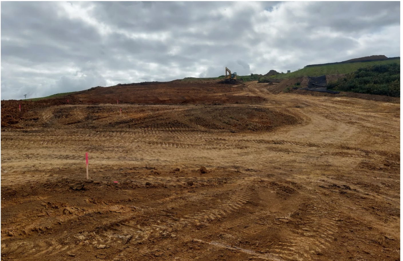
Subgrade near finished level
