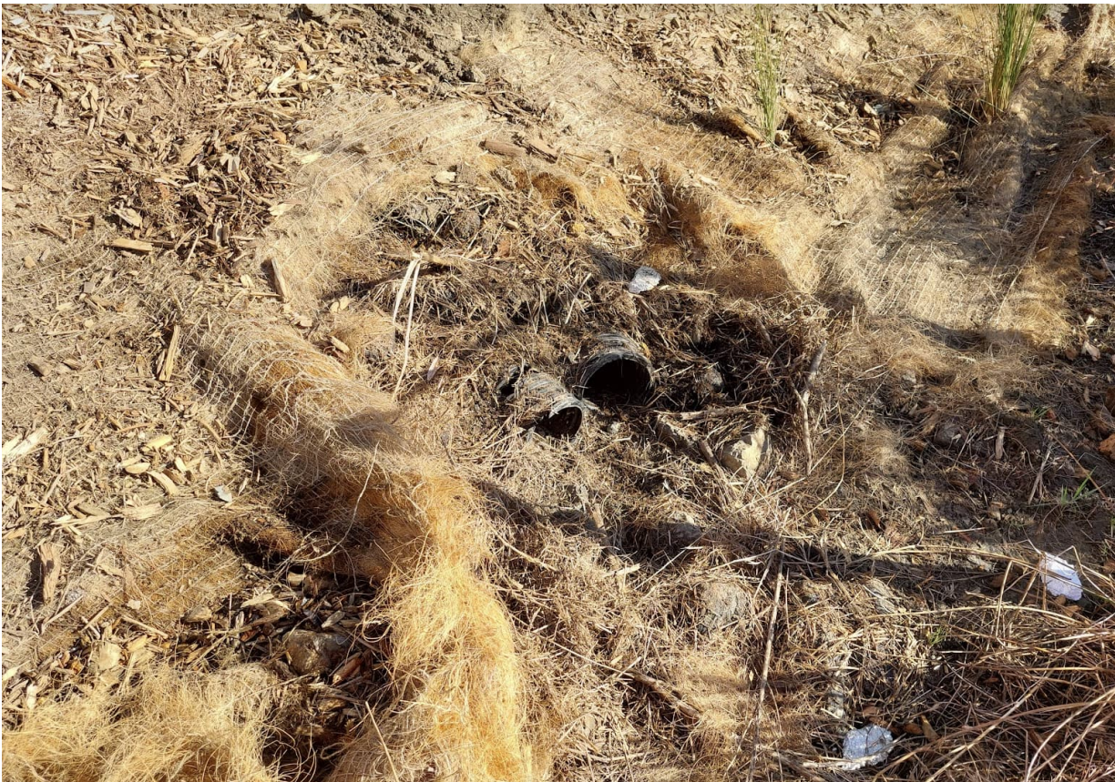
Contractor exposed underfill drain (toe of REB1) that was previously covered in vege mat
